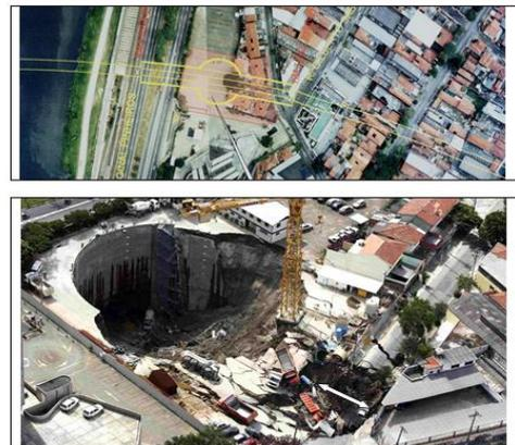
Figure 1. The Pinheiros station cavern and shaft collapse of 12<sup>th</sup> January 2007. The white arrow indicates the axis of the station cavern, and the fallen white car indicates the rear discontinuity.
