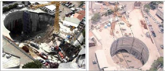
Figure 1. The dramatic cavern collapse in São Paulo, during construction of the Line 4 subway. The feature 'FF' marks the limit of the collapse, in the street Rua Capri, where six people died.
