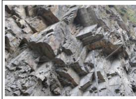
Figure 1. Confronted with this potentially unstable jointed rock slope, multiple reasons for the over-break and instability suggest themselves. There are clearly adverse values of JRC, JCS, and  $\phi$ , and there are also adverse ratings of Jn, Jr, Ja (and Jv on occasion).
