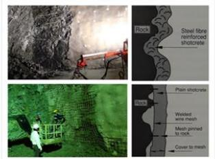
Fig 1. Top: Single shell shotcrete final lining with fibre reinforced shotcrete and pre-excavation grouting to control water inflow consists of an initial 5cm layer of S(fr) and permanent C1-bolts each applied close to the face bottom. Wire mesh reinforcement demonstrates the difficulties caused by overbreak. (Credit: Right images courtesy 'Vandevaele')
