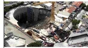
Figure 1. The Pinheiros station cavern and shaft collapse of 12<sup>th</sup> January 2007.
