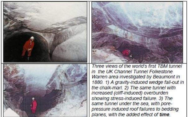
Three views of the world's first TBM tunnel in the UK Channel Tunnel Folkestone Warren area investigated by Beaumont in 1880. 1) A gravity-induced wedge fall-out in the chalk-marl. 2) The same tunnel with increased (cliff-induced) overburden showing stress-induced failure. 3) The same tunnel under the sea, with pore-pressure induced roof failures to bedding planes, with the added effect of time.
