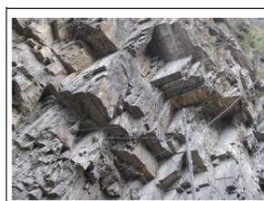
Figure 1. Confronted with this potentially unstable jointed rock slope, multiple reasons for the over-break and instability suggest themselves. There are clearly adverse values of JRC, JCS, and  $\phi$ , and there are also adverse ratings of  $J_n$ ,  $J_r$ ,  $J_o$  (and  $J_w$  on occasion).
