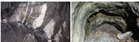
Fig. 1 Chlorite-filled and graphite-coated discontinuities in a Norwegian headrace tunnel, causing over-break, a typical case record for Q-development. Fault-zone and swelling-clay induced failure in Ponte do Pedro, Brazil.
