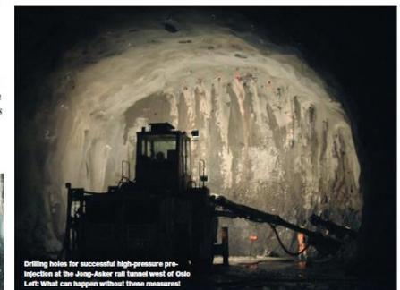
Drilling holes for successful high-pressure pre-injection at the Jung-Ashir rail tunnel west of Oslo. Left: What can happen without these measures.
